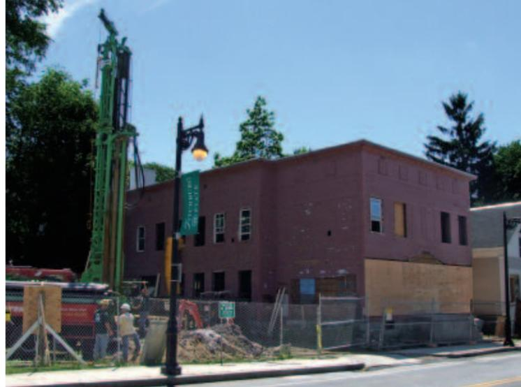
Crews lay the groundwork for a geothermal heating and cooling system for the future Exercise and Sport Science Building on North Street.
